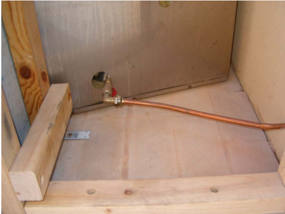
Fitting the Gas Line – 1/2 “ copper
